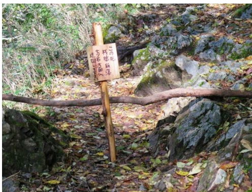
栈橋崩落で通行止めの立て札
